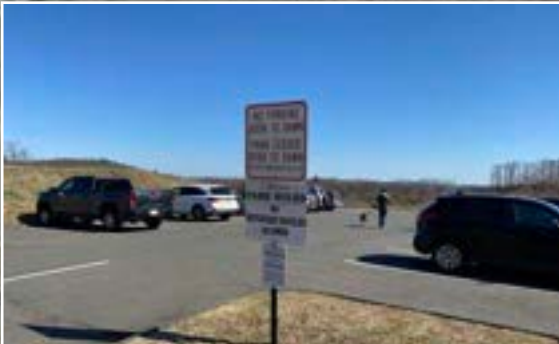
ASPHALT PARKING LOT WITH PARK SIGNAGE
