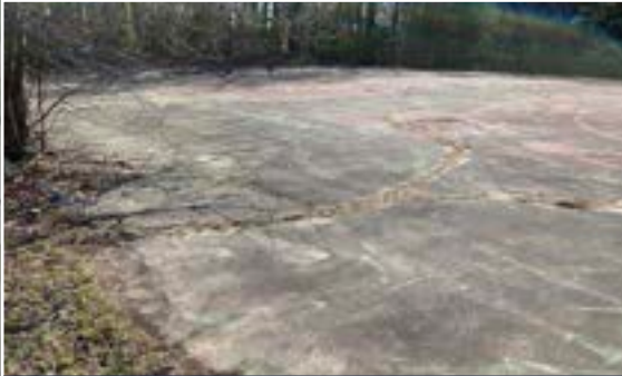
TENNIS COURT HAS SIGNIFICANT CRACKING AND IS IN NEED OF REPAIR
