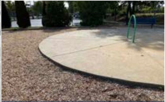
PLAYGROUND REQUIRES ADDITIONAL MULCH
