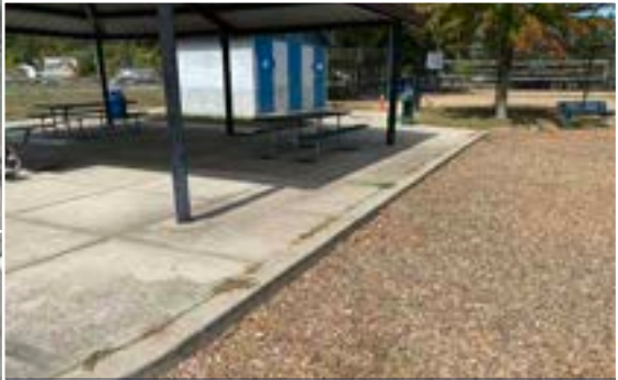
SHADE STRUCTURE AT PICNIC AREA, MULCH ELEVATION IS LOW
