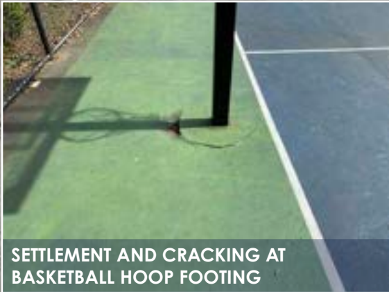
BASKETBALL COURT IS CRACKING AND REQUIRES REPAIR AND RESURFACING
