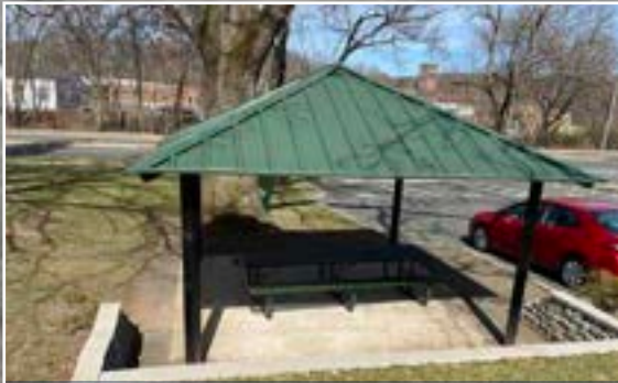
SHADE STRUCTURE WITH SEATING AT PARKING LOT AREA
