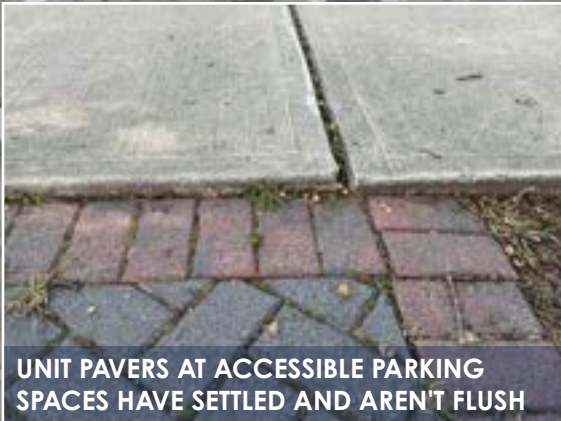
UNIT PAVERS AT ACCESSIBLE PARKING
