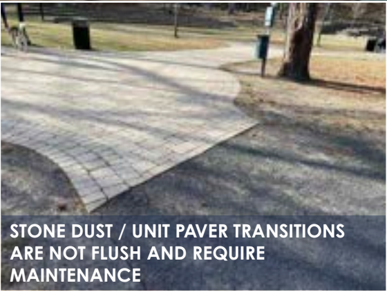
STONE DUST / UNIT PAVER TRANSITIONS ARE NOT FLUSH AND REQUIRE MAINTENANCE
