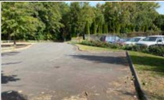
ACCESSIBLE PARKING SPACES DO NOT MEET CURRENT ADAAG REQUIREMENTS
